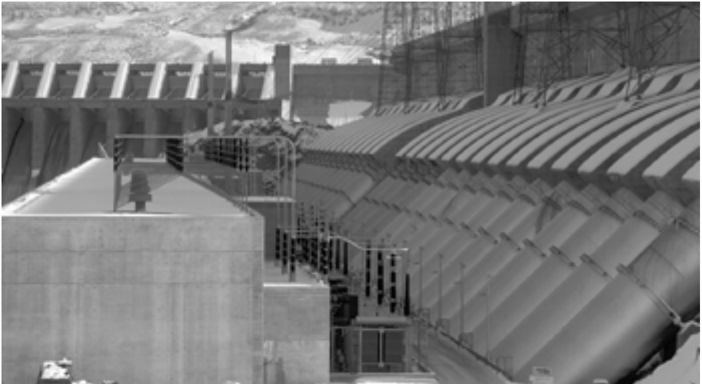
The J. Strom Thurmond Lake and Dam Powerhouse, Clarks Hill, SC, is one of 75 hydropower facilities operated by the U.S. Army Corps of Engineers.
