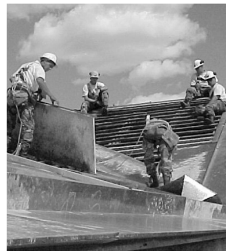
Army engineers repair the roof on a hospital in Mongolia.
