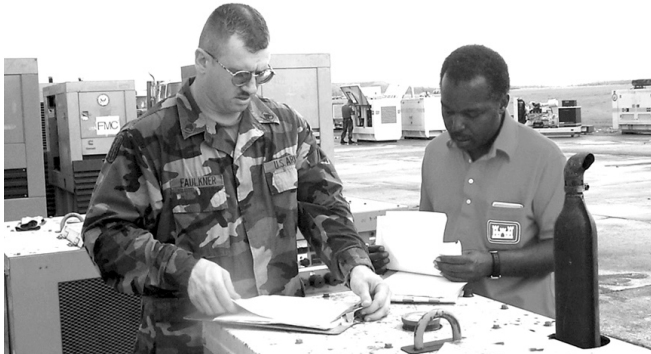
Soldiers and Army civilians from the US Army Corps of Engineers provided emergency power to much of Puerto Rico in the wake of Hurricane Georges.
