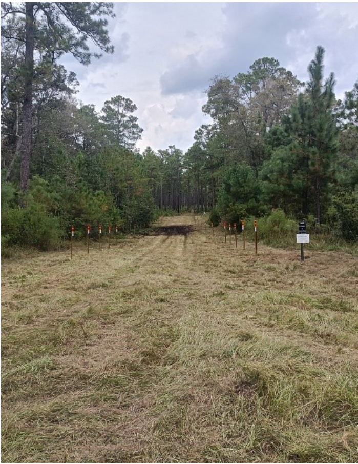
Integrated Training Area Management-constructed low water crossings are sustainable structures which facilitate maneuver through wetlands without precipitating erosion or obstructing the natural course of water. Fort Stewart, Georgia. (Photo Credit: U.S. Army)
